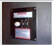
5. Next place the control box in the desired place and mark the 4 mounting holes. Make sure the control box is being mounted in a location that will allow the 2 ft or 10 ft cable to reach the UV tube. Pre drill the 4 holes with a 3/32" or smaller drill bit. Place the box back in place and install the 4 provided stainless steel screws.
