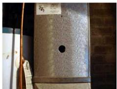
3. Place the UV tube bracket plate over the hole with the black plastic tube mount in the center of the hole with the stickers on the outside as shown. Mark the 4 holes in the corners, Remove the mounting plate and pre drill the 4 holes with a 3/32" or smaller drill bit.
