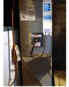
6. Plug the UV cable from the control box into the UV tube. Plug the DC plug from the desktop adapter into the control box. Make sure the power switch is turned off and then plug the desktop adapter into the wall receptacle.
